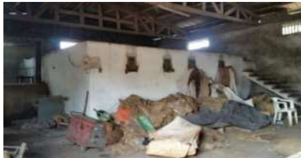
Figure 5: Hybrid solar-electric dryer
